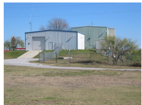
Water Plant located on US Highway 380
