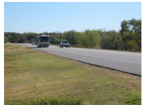
US 380 running basically east-west is an example of freeway classification
